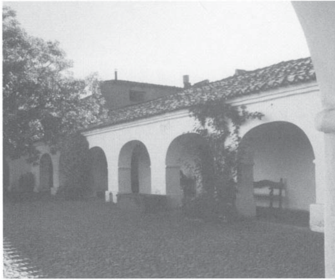
Fig. 15. The Cabildo, Salta, Argentina. Where the sky meets the courtyard, roof tile channels rains, funnels cool night air, and brings a sense of the sky itself into the courtyard.
